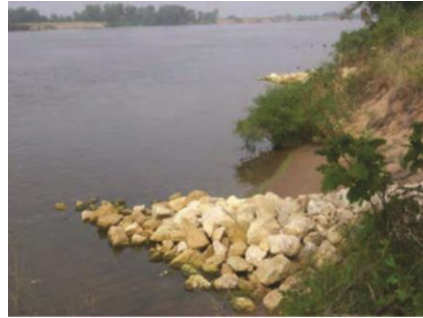
Figure 5.15. Rock vanes at Lost Island Chute, Pool 5, Upper Mississippi River. Photo credit: USACE, Rock Island District.
