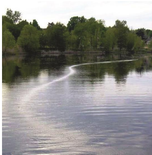
Figure 6.2. Oxygenation with a linear diffuser system. Photo credit: Diversified Pond Supplies LLC, Wapakoneta, Ohio.
