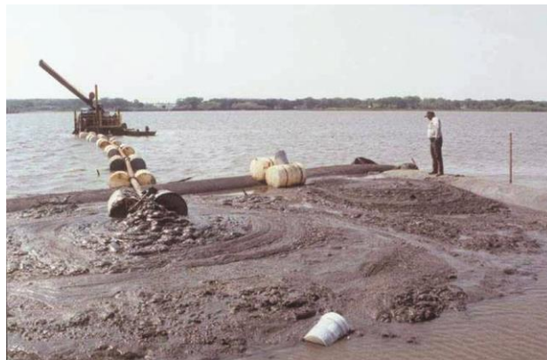
Figure 3.14. The Dry DREdge™ lifts sediment from the reservoir bottom and uses a displacement pump to move it without adding water. The pump fills geotubes with the sediment and then pumps sediment with the consistency of toothpaste behind the tubes to form a small island. Photo credit: J. C. Marlin, Illinois Department of Natural Resources.
