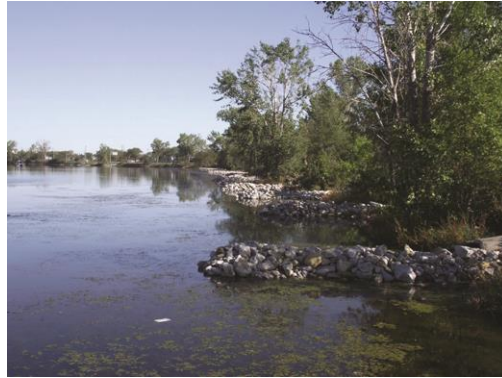
Figure 5.13. Groynes (sometimes referred to as jetties or hardpoints) along a shore of a Nebraska reservoir. Groynes are positioned to reduce nonperpendicular wave energy and allow growth of macrophytes. Photo credit: Nebraska Game and Parks Commission, Lincoln.
