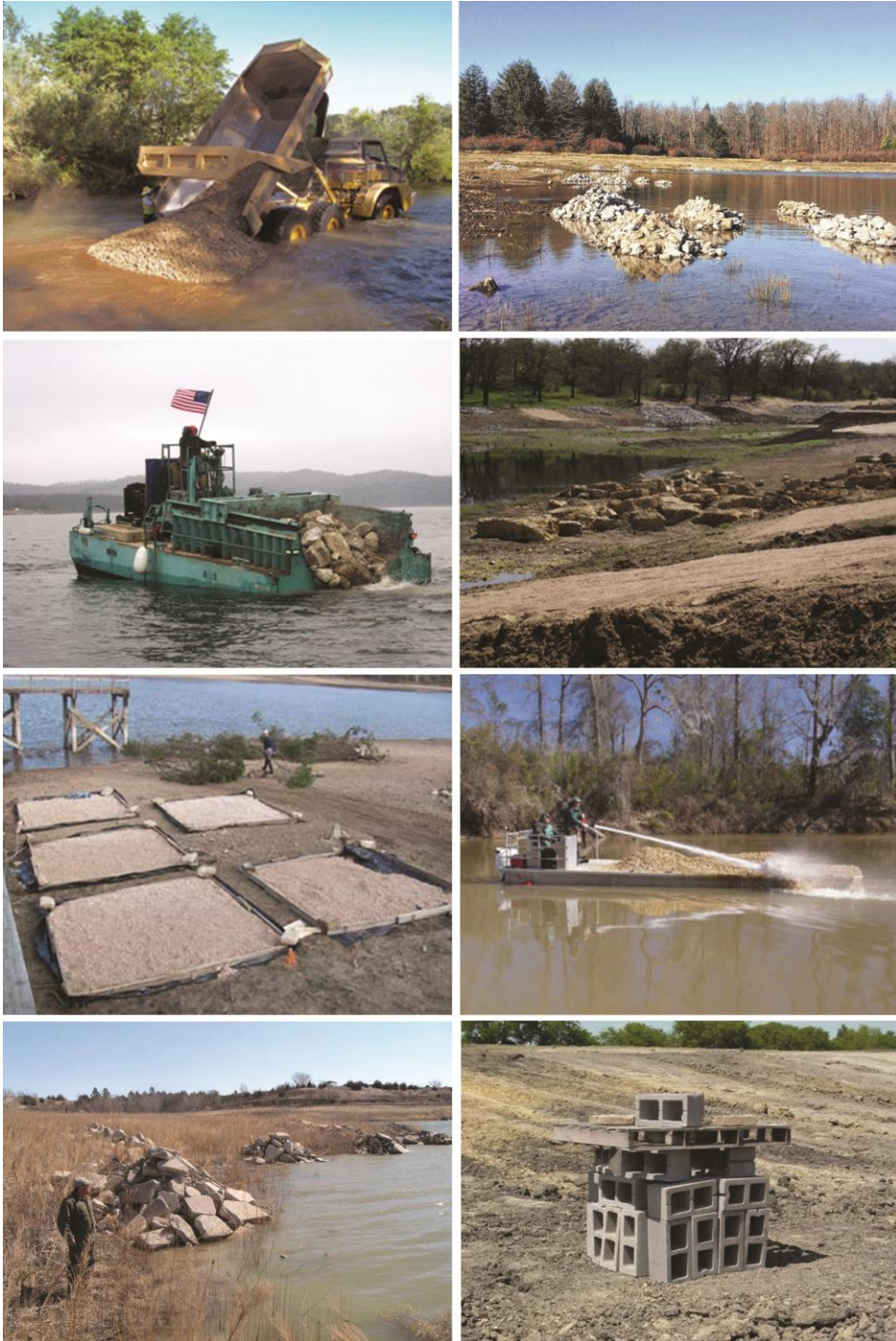
Figure 10.7. Examples of reefs constructed from stone materials. Photo credits: (Left column, top to bottom) FISHBIO, Missouri Department of Conservation, Texas Parks and Wildlife Department, and Nebraska Game and Parks Commission; (Right column, top to bottom) Pennsylvania Fish and Boat Commission (top two), Georgia Department of Natural Resources, and Pond Boss Magazine.
