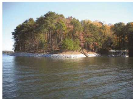
Figure 5.16. Shore revetted with riprap in Lake Lanier reservoir, Georgia, to prevent bank erosion induced by wave action. Photo credit: Marine Specialties, Inc., Gainesville, Georgia.
