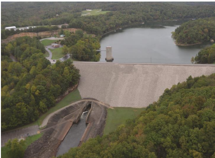
Figure 1.6. Tailrace area immediately below the Nolin Lake dam, Kentucky. Photo credit: U.S. Army Corps of Engineers, Louisville District.
