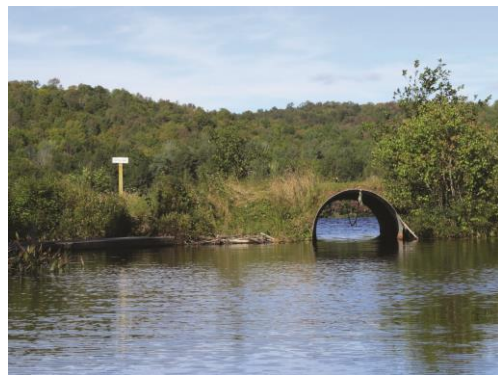
Figure 9.5. Culvert installed on an embankment built across the back of a cove. Photo credit: www.slideshare.com .
