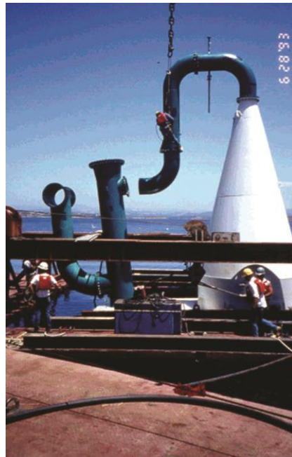
Figure 6.7. Speece cone installation at Camanche Reservoir, California. Photo credit: R. Jung, East Bay Municipal Utility District, Orinda, California.
