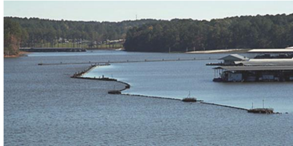
Figure 5.10. View of a floating breakwater, Lake Allatoona reservoir, Georgia. Photo credit: J. Chulick.
