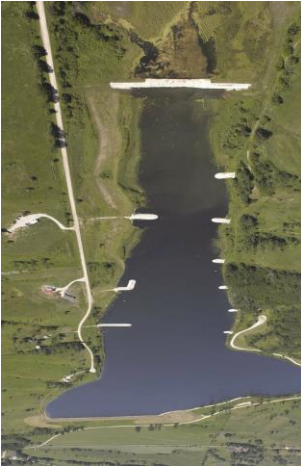
Figure 3.8. A sediment dike (subimpoundment) constructed at the upper end of a Nebraska reservoir. Also shown are groynes and jetties constructed to reduce wind-induced wave action that erodes shorelines. Photo credit: M. Porath, Nebraska Game and Parks Commission, Lincoln.
