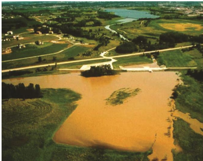
Figure 3.7. Sediment basin constructed above Wehrspann Reservoir, Nebraska, to trap sediment and improve water clarity. Note clear-water reservoir in background. Photo credit: Nebraska Game and Parks Commission, Lincoln.
