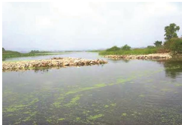
Figure 9.4. Partial closure structure at the Weaver Bottoms secondary channel, Pool 5, Upper Mississippi River. Photo credit: USACE, Rock Island District.
