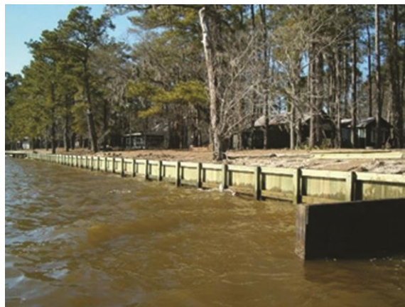
Figure 5.19. Bulkhead designed to control wind-induced shore erosion. Photo credit: M&M Marine Construction, Queenstown, Maryland.
