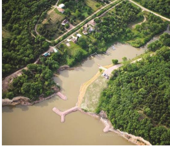
Figure 5.7. Breakwaters positioned at the mouth of an embayment to reduce wind-induced wave action originating in the reservoir. Photo credit: M. Porath, Nebraska Game and Parks Commission, Lincoln.
