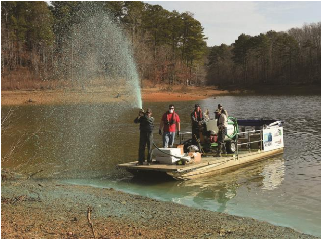
Figure 11.14. A team of Alabama Power and U.S. Forest Service biologists used a pontoon boat equipped with a spray rig and 150-gallon tank to hydroseed banks of Smith Lake reservoir, Alabama. Photo credit: Alabama Power, Birmingham.
