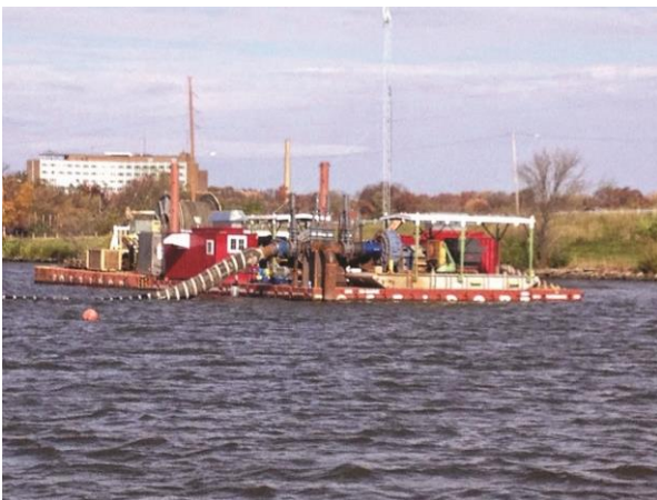
Figure 3.12. Hydraulic dredging at Decatur Lake, Illinois, part of a $91 million reservoir restoration. Photo credit: M. Honnold, Macon County, Illinois.
