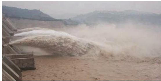
Figure 3.9. Sediment sluicing through a dam in the Yellow River, China. Photo credit: china.org.cn.
