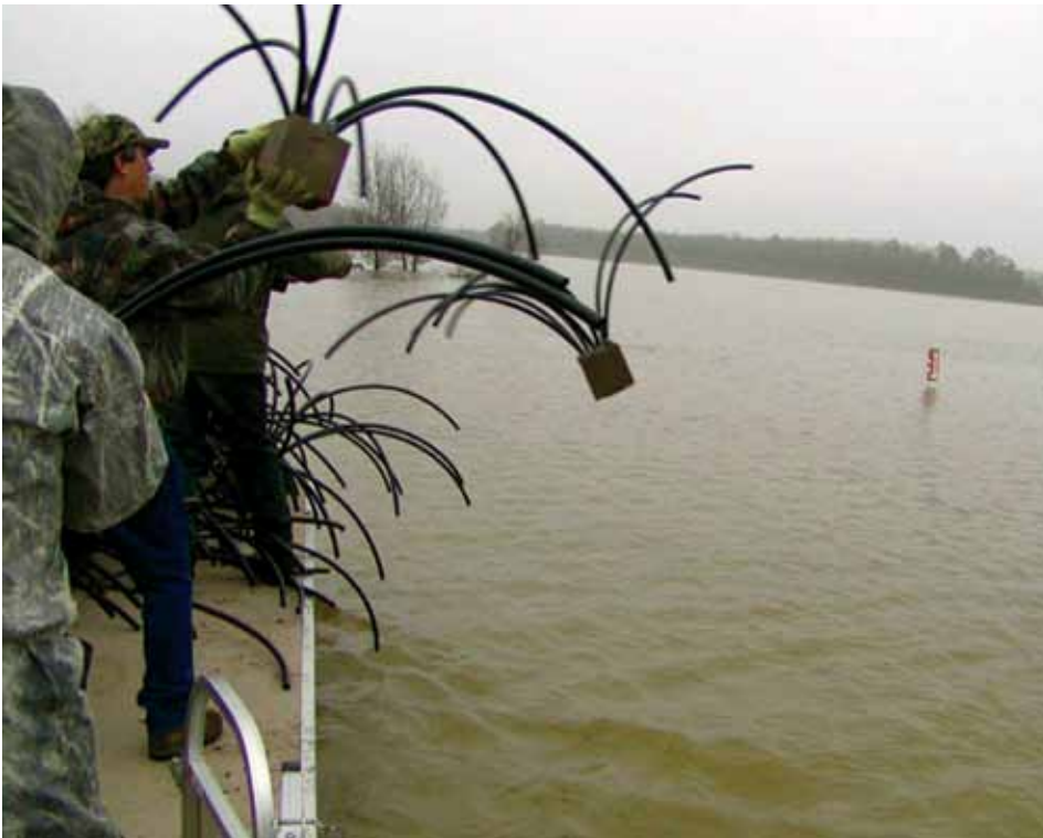
Figure 8. Installing artificial fish habitat in Pine Creek Lake, Oklahoma (source: Oklahoma Department of Wildlife Conservation).
