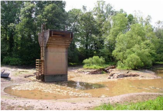
e. Reservoir sedimentation is beginning to bury the outlet works at Deep Creek Dam, NC, 2007.
