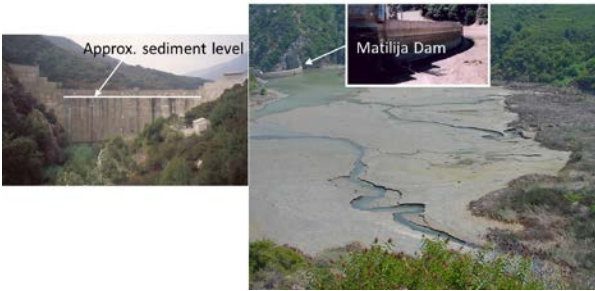
j. Sedimentation has almost completely filled the reservoir behind Matilija Dam near Ventura, CA.
