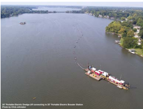
r. Example hydraulic dredging of Lake Decatur reservoir near Decatur, IL (photograph courtesy of GLDD Marketing Department).
