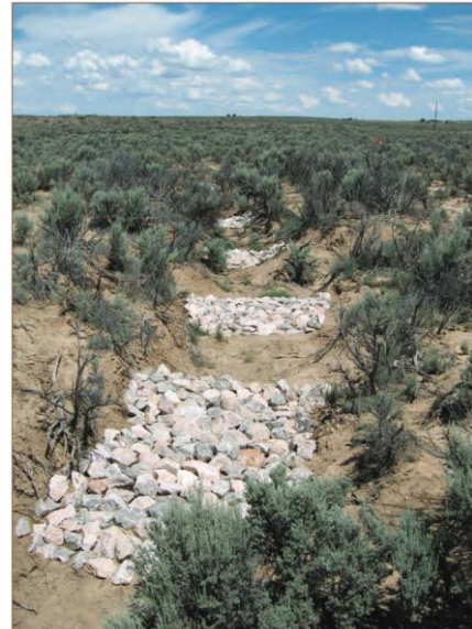
Figure 11. Erosion-control structures in the Penistaja Arroyo drainage. A, July 24, 2009, near the start of the study period. B, July 2, 2013, after completion of the study.
